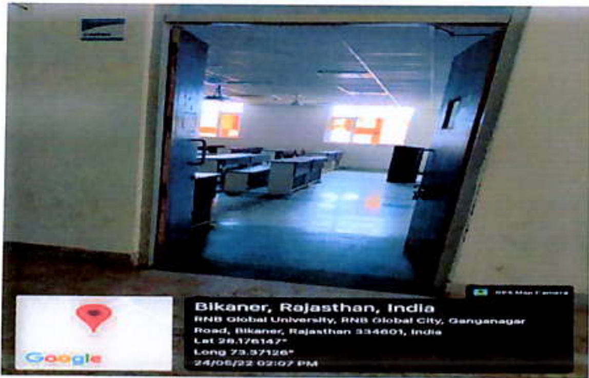
Second Floor Room No. – 212 Classroom front
