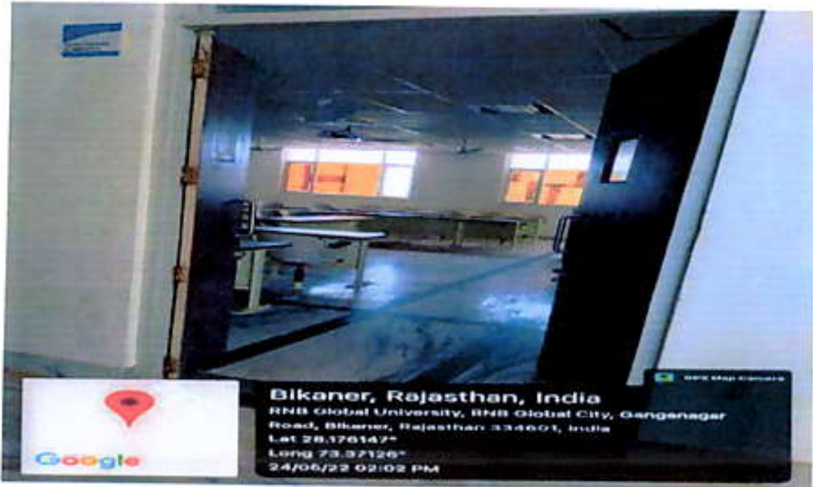
Second Floor Room No. - 213 Classroom front
