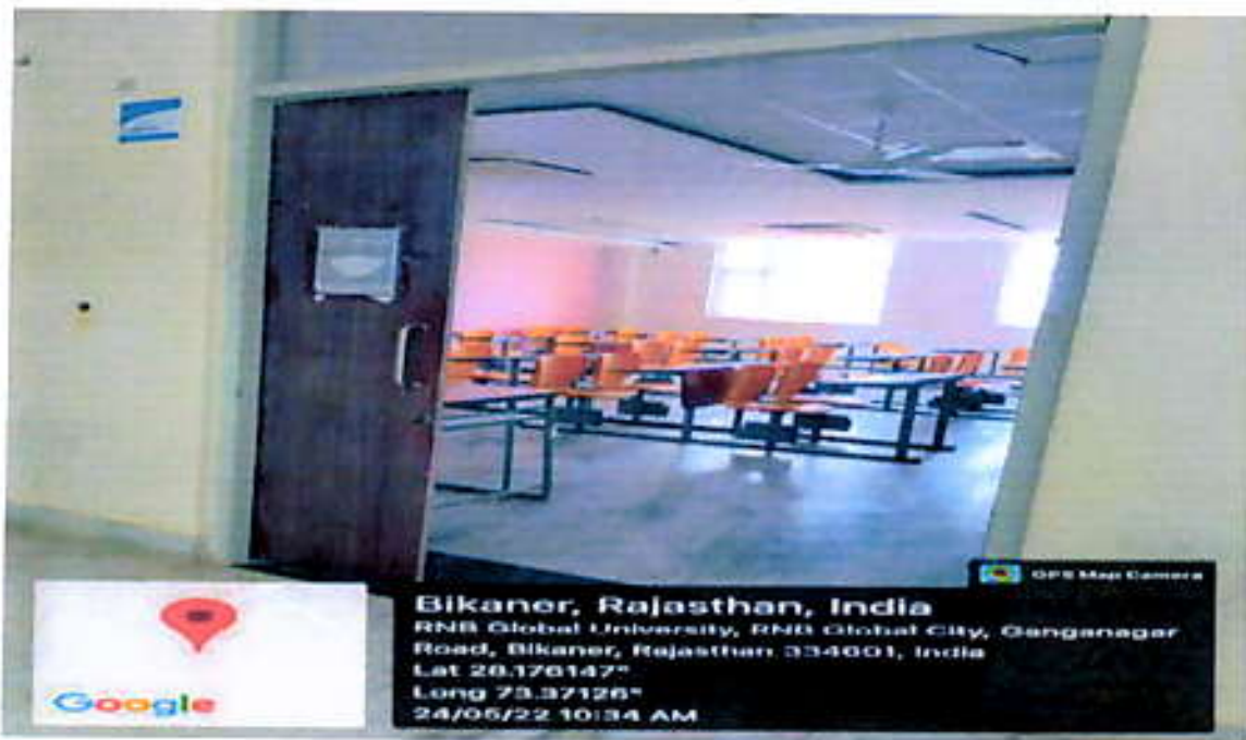
First Floor Room No. 101 Classroom front
