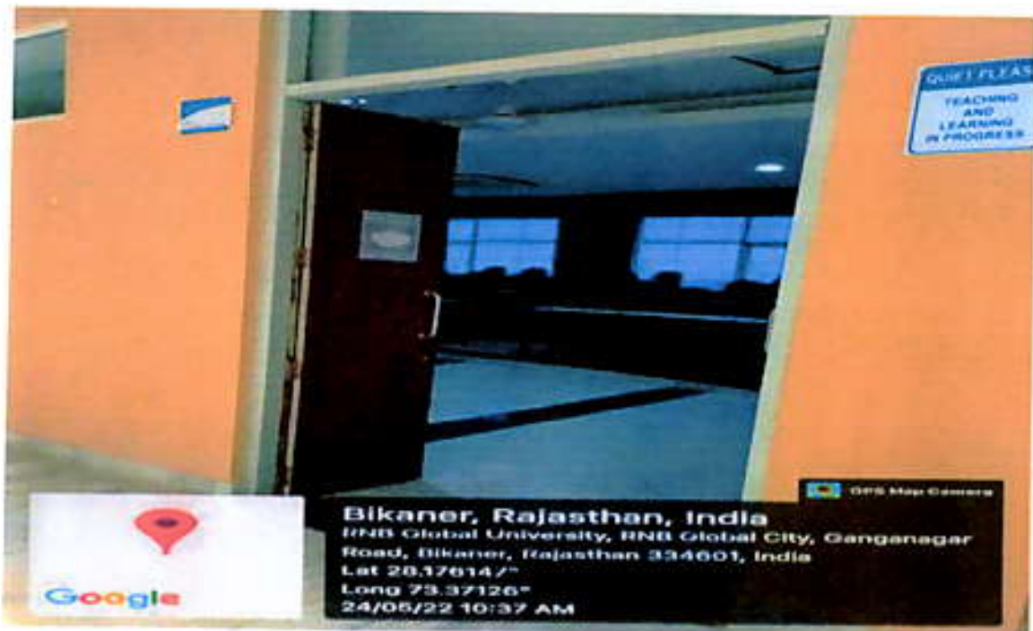
First Floor Room No. 107 Classroom front
