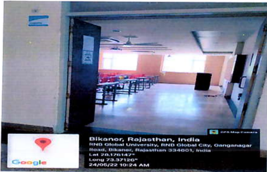
Ground Floor Room No. 001 Classroom front
